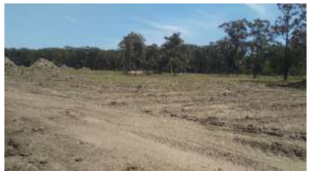
Photograph 10: Facing west from north-eastern corner of site.
